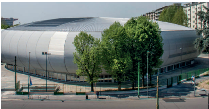
DRAINPANEL Allianz Cloud Sport Hall MILANO, ITALIA
